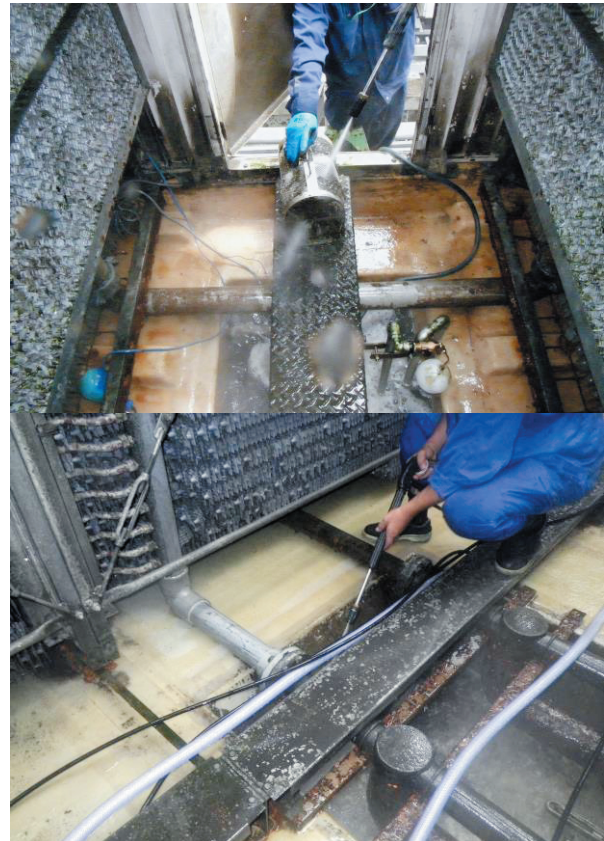
Photograph of the Cleaning the cooling towers
